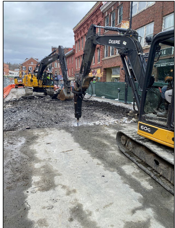
Hebert Excavation removing the roadway on State Street.
